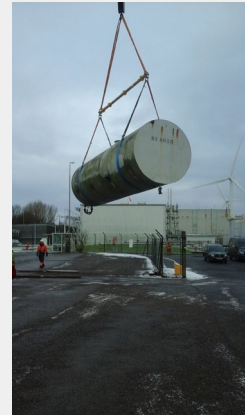
Removing the diesel storage tank
