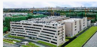
Ningbo Campus II Biologics CDMO 350,000 ft 2
