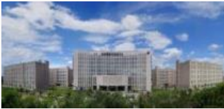
Beijing HQ Laboratory services 1.2 million ft 2
