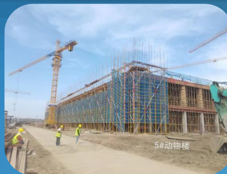
Ningbo Campus III (ongoing construction)
